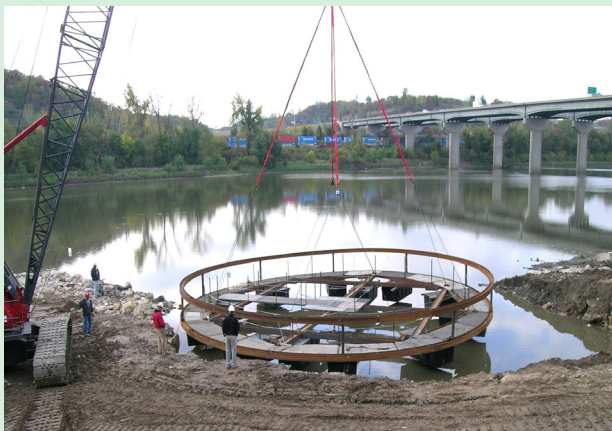
The first of 18 circular cells, 54.5 ft. in diameter on the Kansas River.
