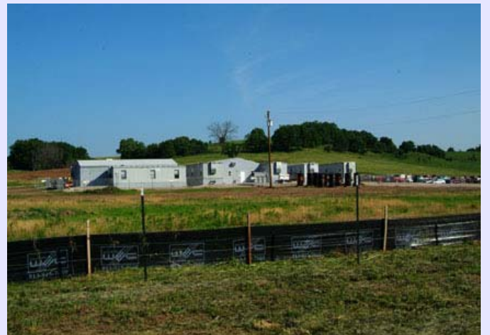
Temporary construction offices are located at the site of the new treatment facilities.
