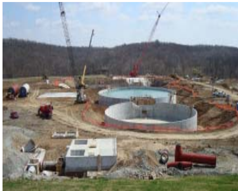
Photo showing contact basins for future water treatment.
